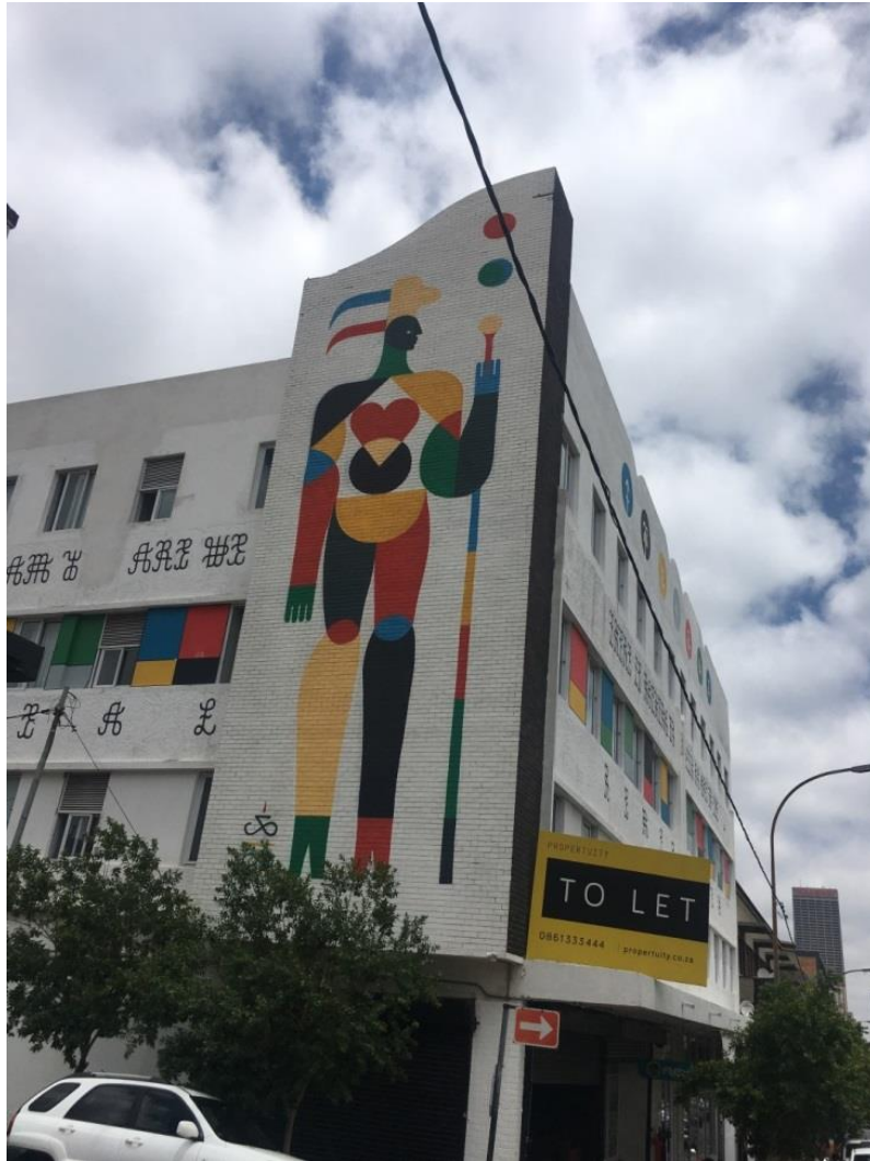
Figure 6.6 Remed's View building.
