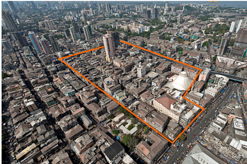
Aerial view of the 16.5-acre area selected for redevelopment in Bhendi Bazaar
